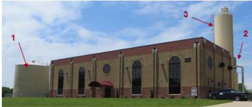
Image 1: CTPWD's (1)-Ground Storage Tank, (2)-Head Tank, and (3)-Lime Silo
